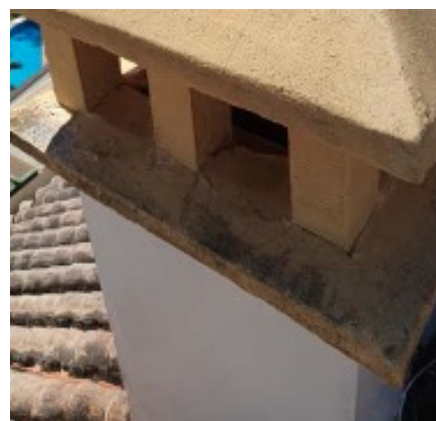
If left to Meridional repairs to the roof would have cost €8,300 plus 10% IVA. The Presidents approach has so far cost €580.00 including IVA!
